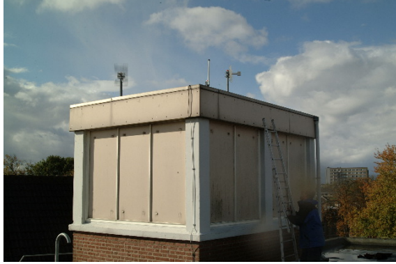
Figure 3: Antennas on a building.
